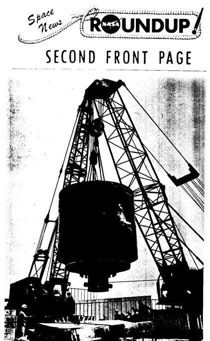
CENTRIFUGE MOTOR PART\_\_Workmen use a heavy duty crane to lift the 197,000 pound rotor for the direct current drive motor which will propel the centrifuge now under construction in the space. Flight Acceleration Facility (Building 34). Delivery was made last week on this part of the largest DC motor ever built which develops 10,700 horsepower. The centrifuge will be capable of generating 30 g's of force on material and lower forces for personnel.
