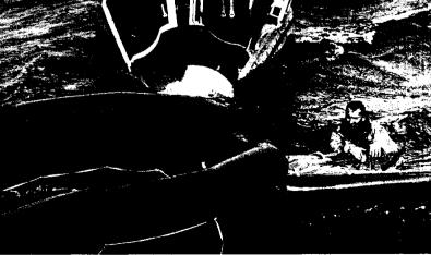
ROUGH WATER RECOVERY --- The Rendezvous and Recovery section of a boilerplate version of the Gemini spacecraft is completely awash during rough water egress tests in the Gulf of Mexico. Astronaut James A. Lovell Jr., one of the test participants is in the water with waves running six to eight feet high.
