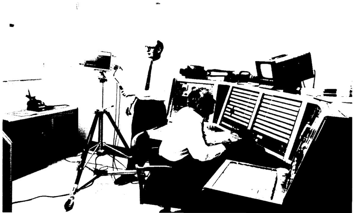
TEACHER'S DESK—Ed Middleton, head of the Cockpit Familiarization Group, mans the instructor's console from which switch positioning and other command module crew actions can be monitored. Sam Wenneker focuses the television camera on a schematic of the command module instrument panel which is fed to the rendezvous window monitors.
