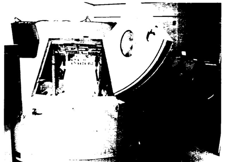
COZY CLASSROOM—It doesn't look much like an Apollo command module from the outside; the cockpit interior accurately depicts for flight controllers the instrument panel and work station layouts. Television monitors are mounted in the rendezvous windows above each student's head to carry the video portion of the instructor's lecture. The audio portion is fed through individual headsets.
