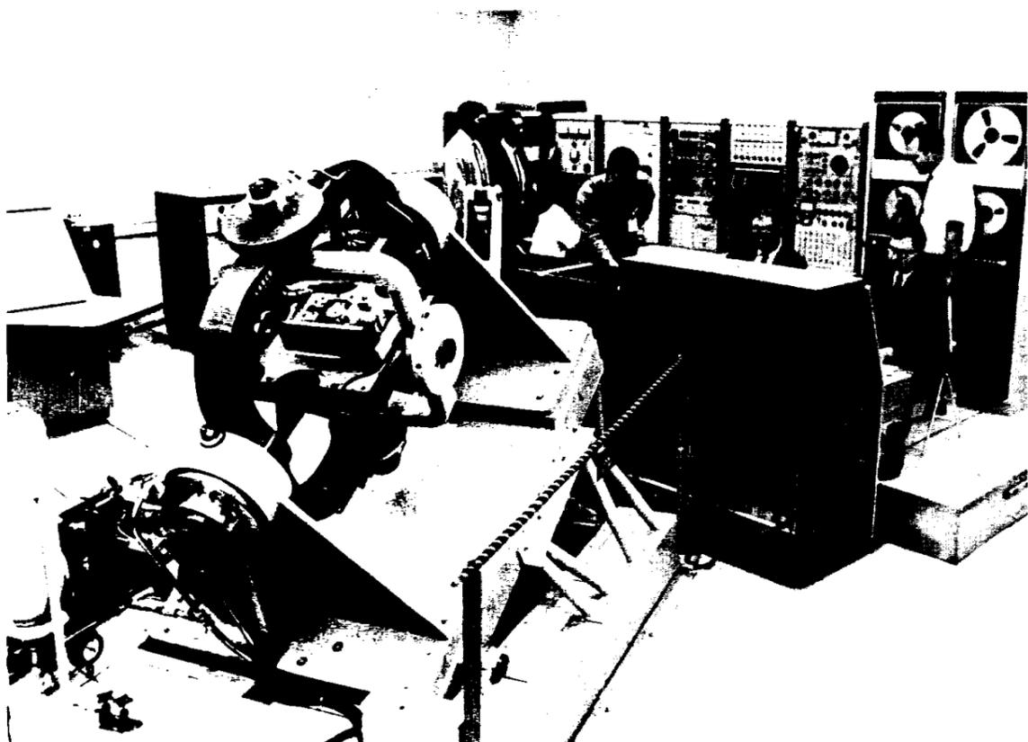
**HEART OF THE MATTER**—The Apollo inertial platform of the spacecraft's stabilization and control system is mounted in the Guidance and Control Laboratory's three-axis servo-controlled simulator in Building 16. Computer-programmed attitude changes by the platform remotely initiated RCS thruster quad firings in the Auxiliary Propulsion Test Facility a mile away.
