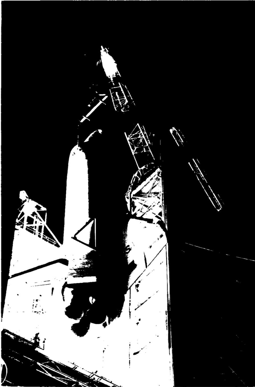
**NIGHTWORK**—Shuttle Orbiter *Enterprise* is hoisted into an unfamiliar position at Marshall Space Flight Center April 21 during preparations for Orbiter/external tank vibe tests later this month. *Enterprise* was hoisted into a test fixture originally built for Saturn V structural testing.
