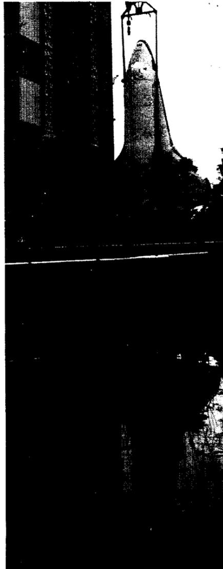
**TWIN ORBITERS**—Orbiter *Enterprise* appears to have a twin as it is hoisted from Marshall Space Flight Center's dynamic test stand. After structural mods to the stand, *Enterprise* will again be lifted into the facility for all-up vibroacoustic tests with the booster.
