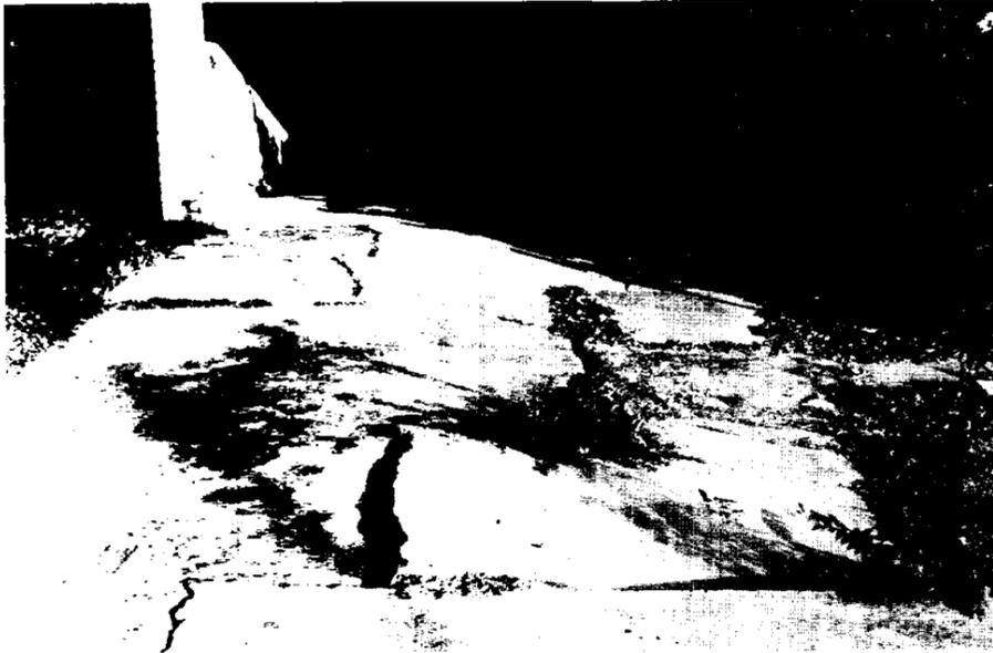
**SHIFTING EARTH**—Surface faults in the Houston area sometimes cause extensive damage to houses and commercial buildings such as this cracked driveway and distorted house on Billings Street. A homeowner with damage from surface faulting is usually stuck with an unsaleable or greatly devalued house.
