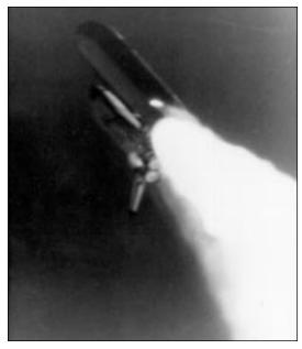
This photograph of 51-L shows the flame developing near the O-Ring on the solid rocket booster. Moments later the entire craft exploded in a fiery ball.
