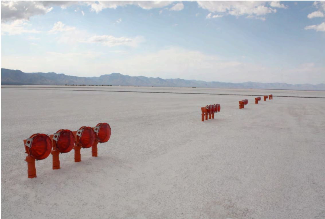
Figure 15A. View of Inner Glide Slope (IGS) Indicator Ball/Bar Lights on Runway 17/35, looking West towards San Andres Mountain Range, 2011.
