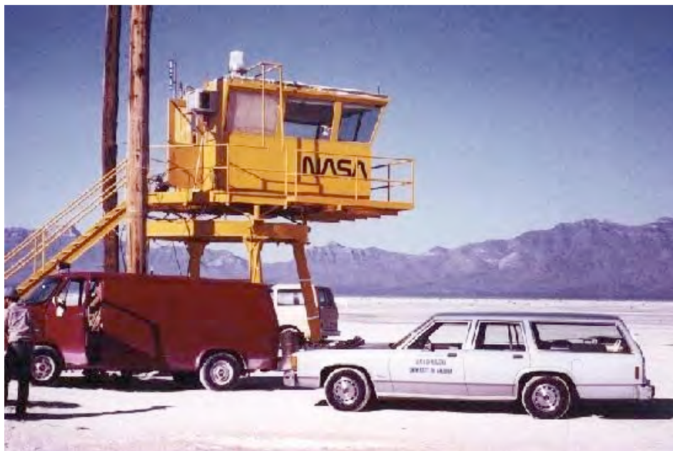
Figure 11A. View of Control Tower, looking northwest, after the cantilevered observation walkway was added, ca.1982 (Source: NASA WSTF).
