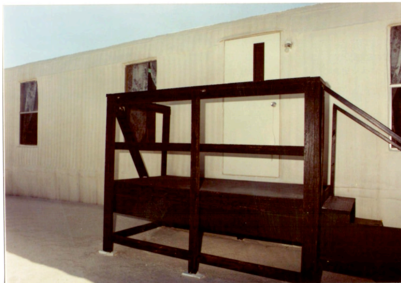
Figure 6B. View of the HUB Maintenance Building, 1988, looking northeast at the trailer wing (Source: NASA WSTF).
