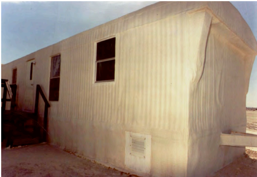
Figure 5B. View of the HUB Maintenance Building, 1988, looking northeast at the trailer wing (Source: NASA WSTF).
