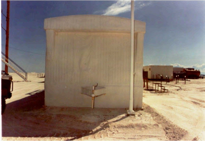
Figure 6A. View of the HUB Maintenance Building, 1988, looking north at the trailer wing (Source: NASA WSTF).
