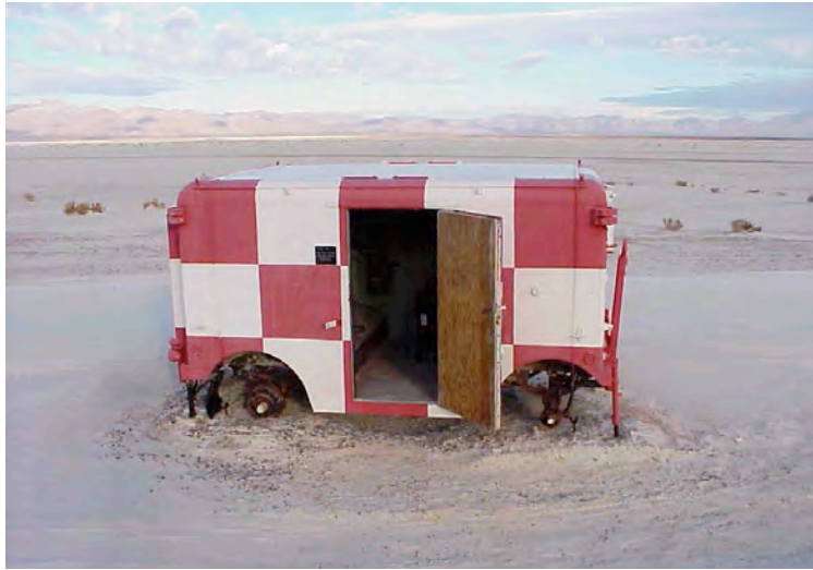
Figure 4A. View of the original PAPI Control Building, looking East with Sacramento Mountain Range in background; this repurposed trailer was replaced around 1992 with the current PAPI Control Building, undated (Source: NASA WSTF).
