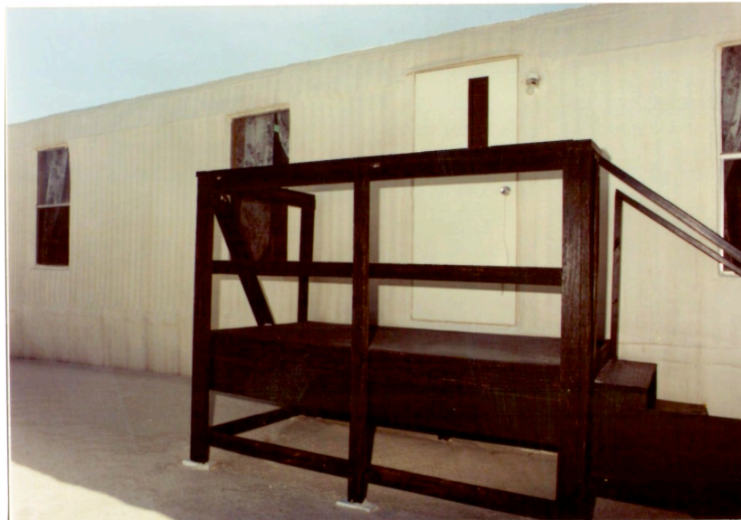
Figure 6B. View of the HUB Maintenance Building, 1988, looking northeast at the trailer wing (Source: NASA WSTF).
