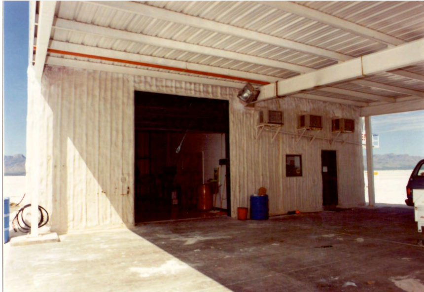
Figure 7A. View of the HUB Maintenance Building, 1988, looking southwest from the carport (Source: NASA WSTF).
