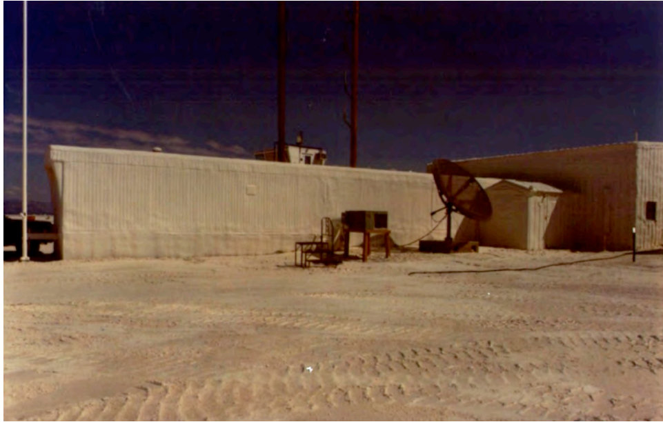
Figure 5A. View of the HUB Maintenance Building, 1988, looking northwest (Source: NASA WSTF).
