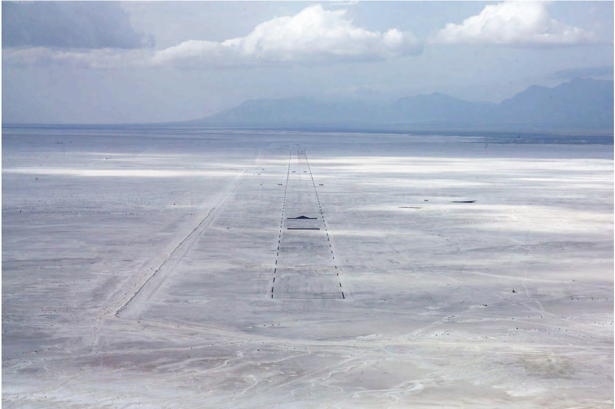
Figure 10. Aerial view of Runway 17/35, looking South towards the San Andres Mountain Range, April 2007 (Source: NASA WSTF).
