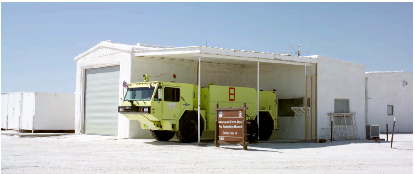
Figure 6B. View of Fire Station No. 4, 2003, looking southeast (Source: NASA WSTF).
