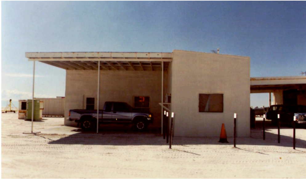
Figure 5A. View of Fire Station No. 4, 1988, looking east (Source: NASA WSTF).
