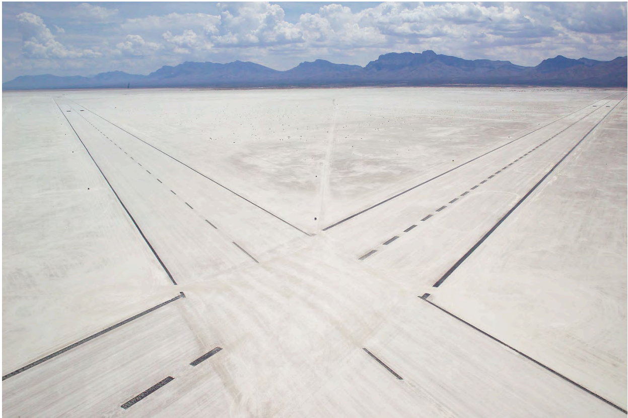
Figure 10. Aerial view of Intersection of Runways 17/35 and 23/05, looking West towards the San Andres Mountain Range, June 2006 (Source: NASA WSTF).
