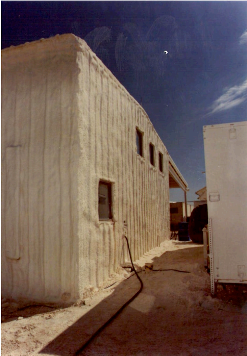
Figure 8. View of the HUB Maintenance Building, 1988, looking north (Source: NASA WSTF).
