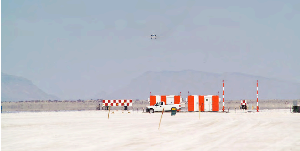
Figure 3. View of Microwave Scanning Beam Landing System Ground Station and Xenon Light Trailer at north end of Runway 17/35, looking northwest, during training exercise in 2010 (Source: NASA WSTF).
