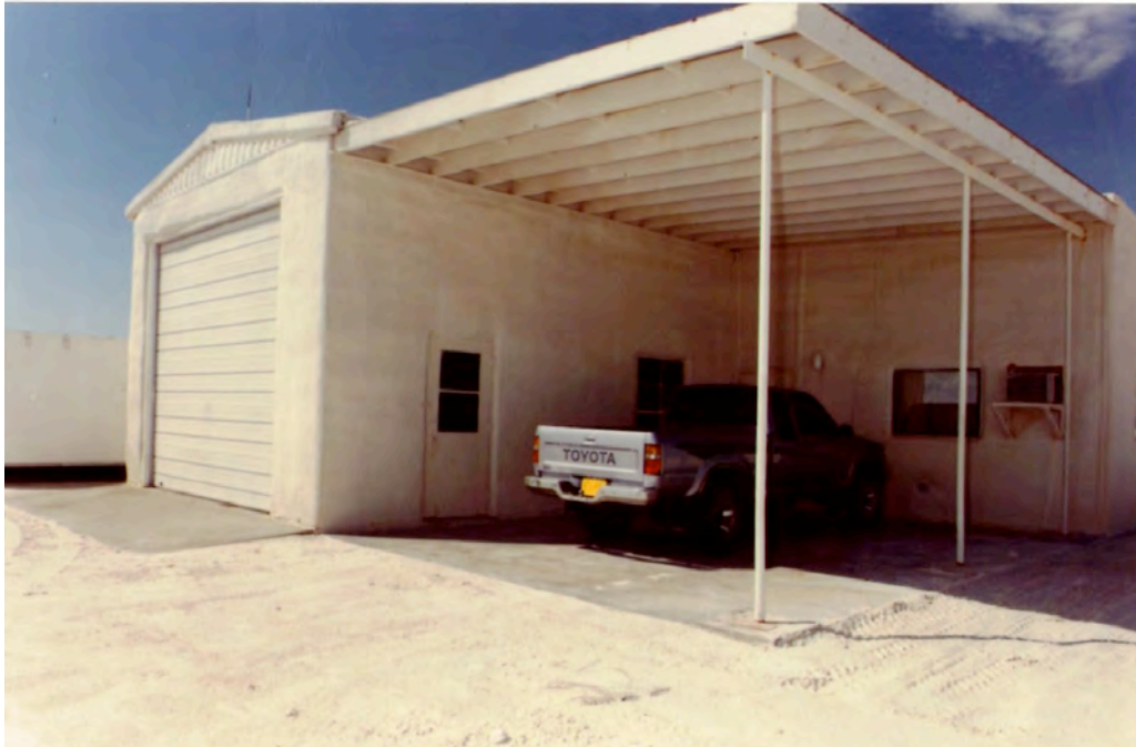
Figure 6A. View of Fire Station No. 4, 1988, looking southeast (Source: NASA WSTF).
