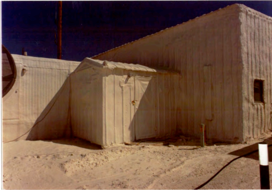
Figure 6. View of the HUB Generator Building, 1988, looking northwest (Source: NASA WSTF).
