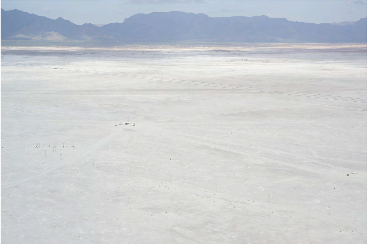
Figure 3. Aerial View of HUB Complex, looking West towards the San Andres Mountains, 2007 (Source: NASA WSTF).
