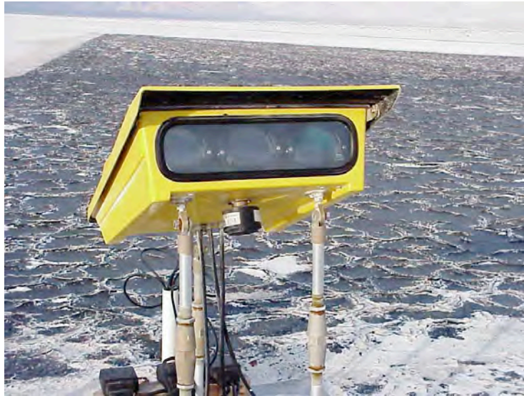
Figure 3A. View of an individual PAPI housing assembly at north end of Runway 23/05, looking west with the San Andres Mountain Range in background, ca.2005 (Source: NASA WSTF).
