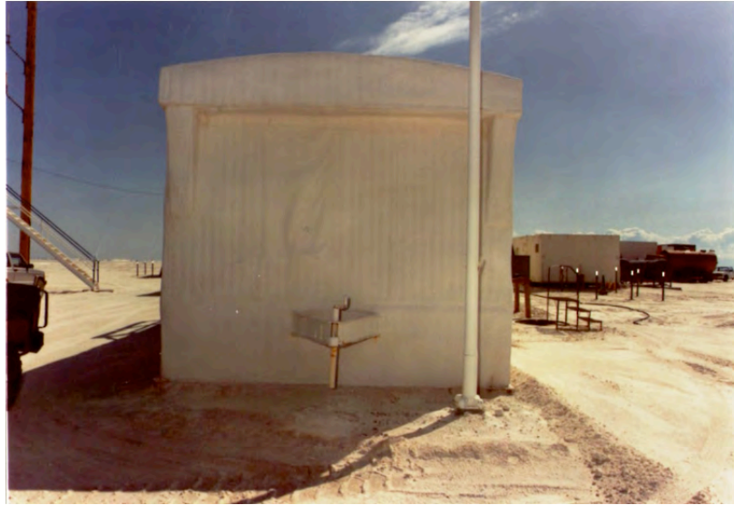
Figure 6A. View of the HUB Maintenance Building, 1988, looking north at the trailer wing (Source: NASA WSTF).
