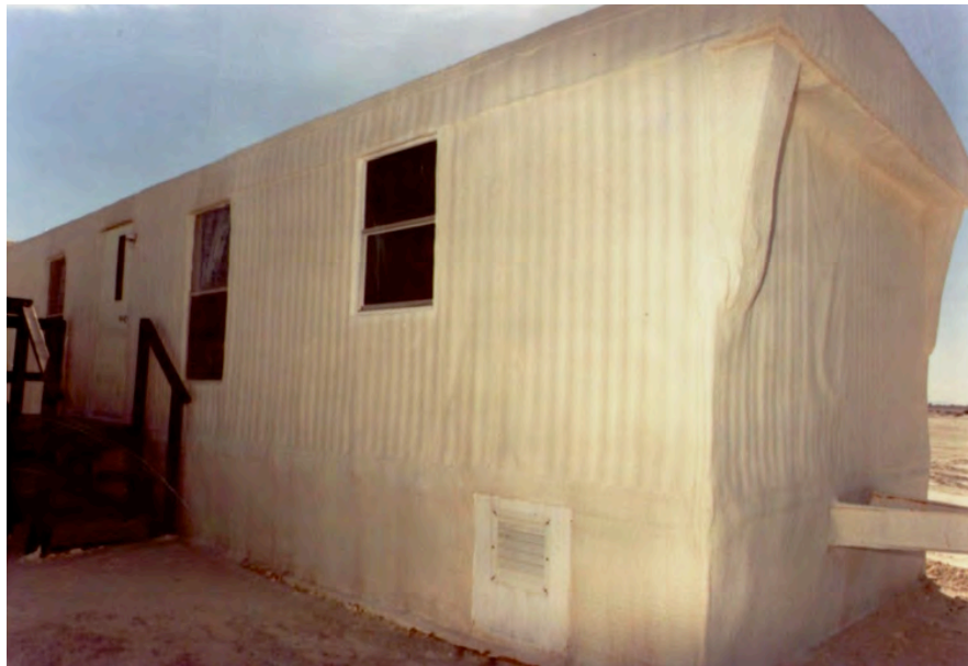
Figure 5B. View of the HUB Maintenance Building, 1988, looking northeast at the trailer wing (Source: NASA WSTF).
