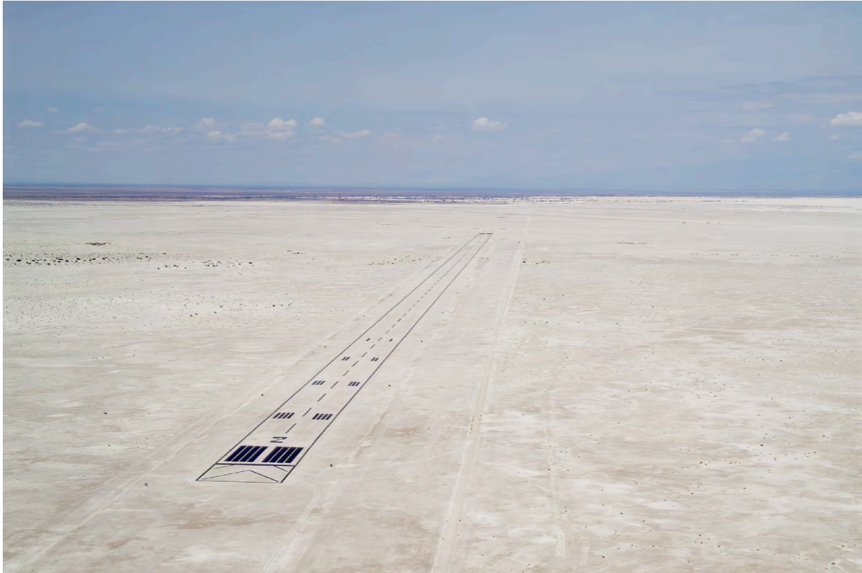
Figure 7. Aerial view of Runway 20/02, looking North towards the Sacramento Mountains, 2006 (Source: NASA WSTF).
