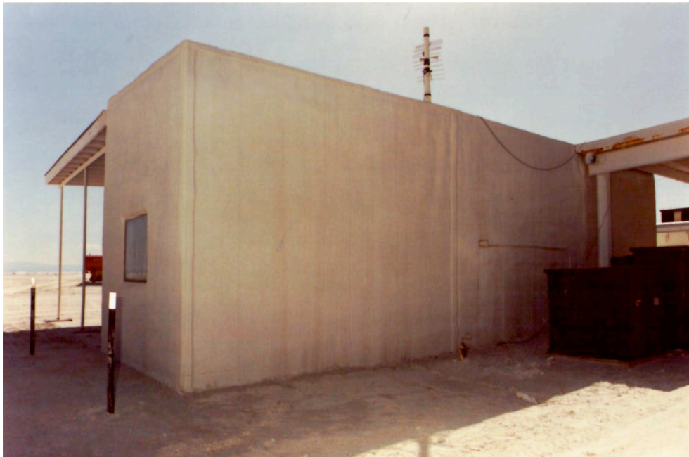
Figure 5B. View of Fire Station No. 4, 1988, looking northeast (Source: NASA WSTF).
