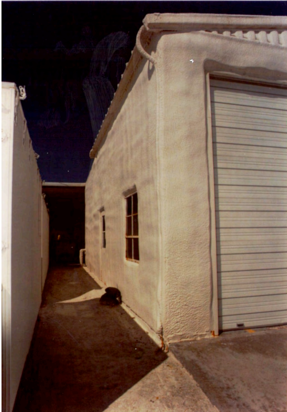
Figure 4. View of Fire Station No. 4, 1988, looking southwest (Source: NASA WSTF).
