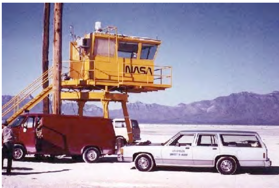
Figure 11A. View of Control Tower, looking northwest, after the cantilevered observation walkway was added, ca.1982 (Source: NASA WSTF).
